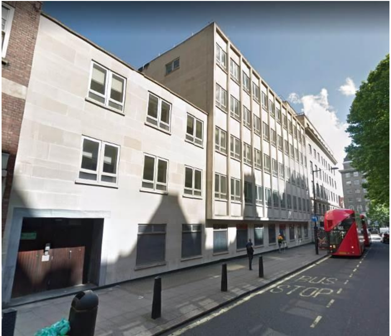
Application site as seen from Great Central Street
